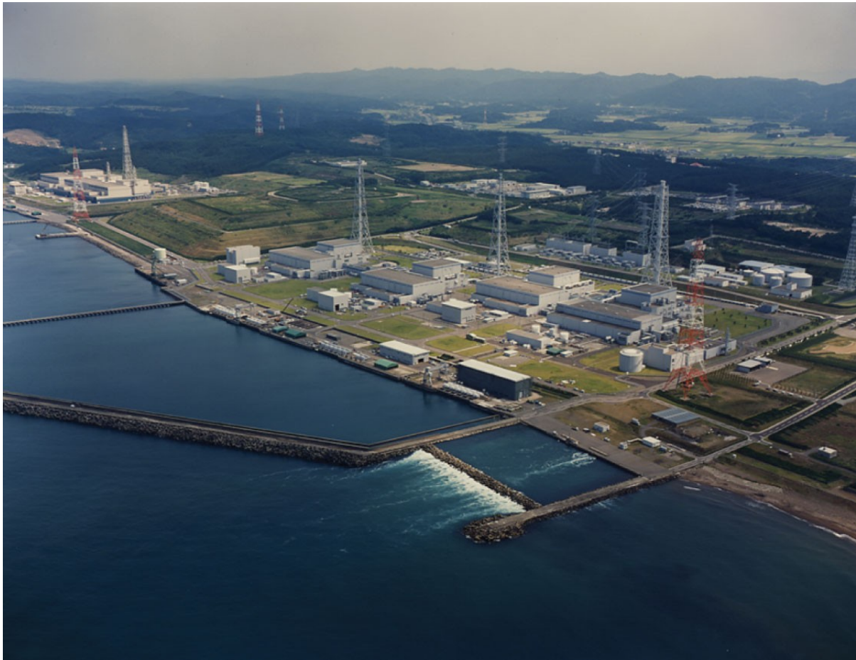
Kashiwazaki - Kariwa Nuclear Power Station
