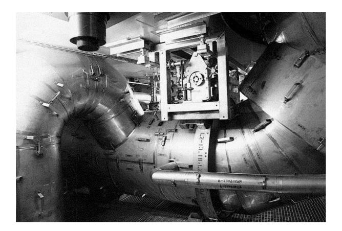
Figure 4: Main coolant pipe inspection rails
