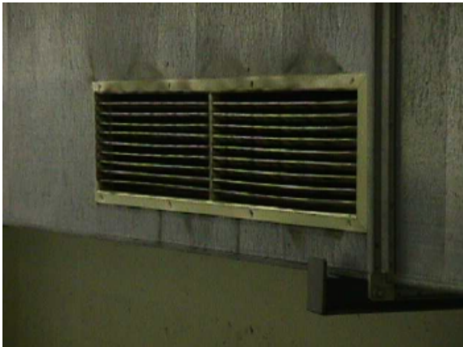
Picture 17 Deposit of Dust at the Exhaustion of Ventilation Installations.
