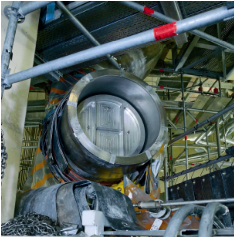
Figure 6: Decontaminated and sealed part of the loop (closure leg)
