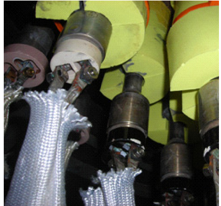
PZR Heater Penetration Sleeve Shields
