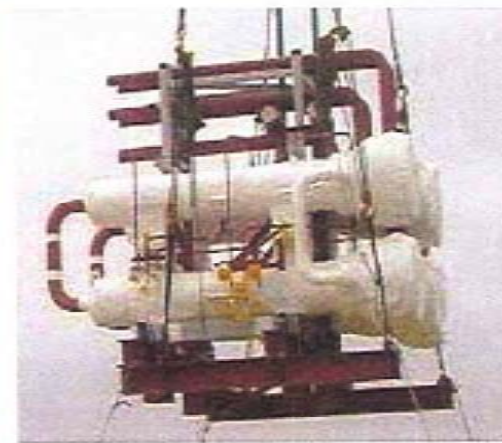
CUW Reheat Exchanger Module
