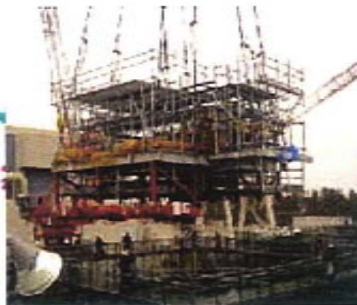
Piping Unit in T-G Pedestal Module
