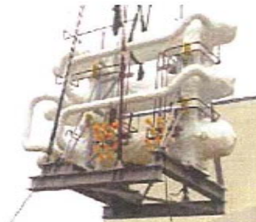
CUW Heat Exchanger Module
