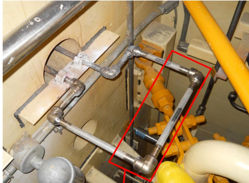
**New Jumper to Bypass the Delay Coils**
