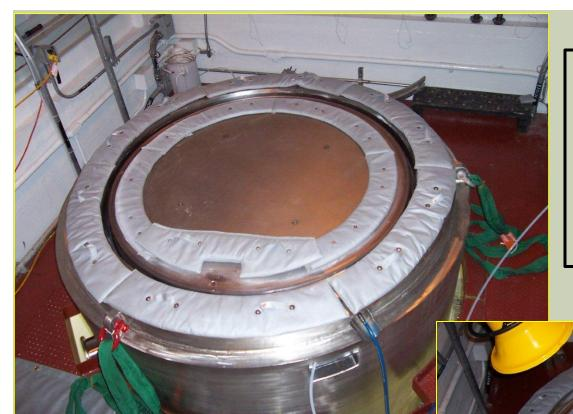
Moveable Lead Shielding to Reduce Gamma Exposure
