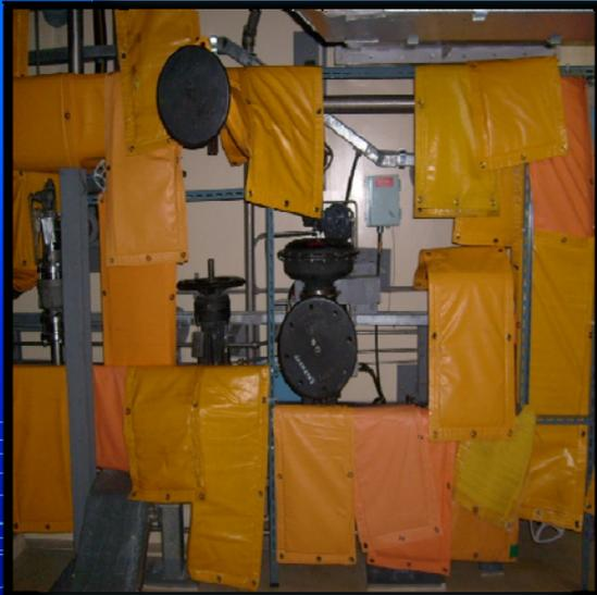
Install direct radiation shield
