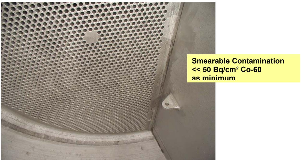
**Figure 3:** SG channel head surfaces with tube sheet after decontamination
