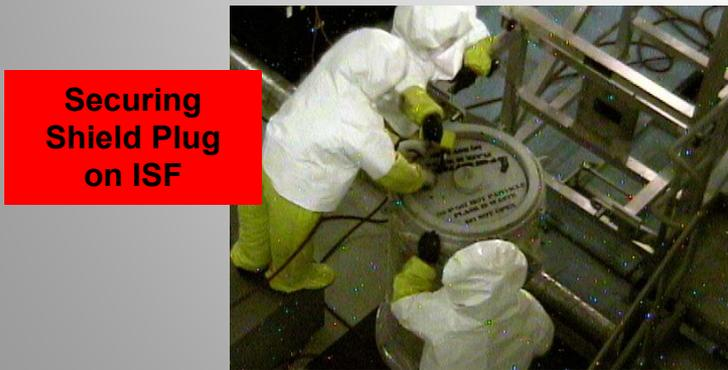
Securing Shield Plug on ISF
