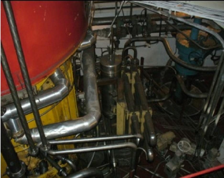
1. Decrease of gamma dose rate from sealing water pipes (presence of high radioactive point sources in the pipes gave dose rate around 10-100 mSv/h).
