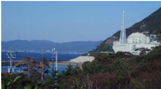
The prototype FBR Monju has an output of 280 MW electrical. It achieved initial criticality in April 1994. In August 1995, Monju became the first Japanese FBR to generate power. It remains the only Japanese facility that can generate electricity using a fast breeder reactor. In December 1995, sodium coolant leaked from a temperature sensor in the secondary system piping. Since then, plant operation has been suspended.
