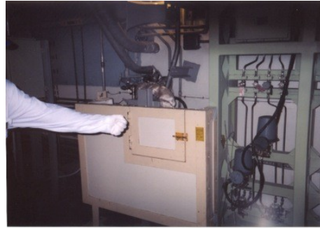
Fixed biological shielding with an access hatch for checking a valve at Almaraz NPP
