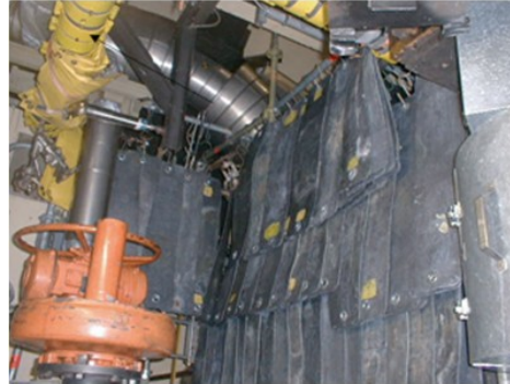
“Bracelet” type protection on a pipe
