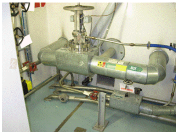
P3: CVCS - Non regenerative heat exchanger
