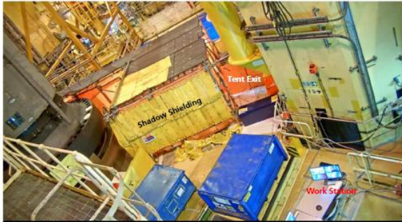
Overview of tent showing tent exit and location of EDM/Inspection work station
