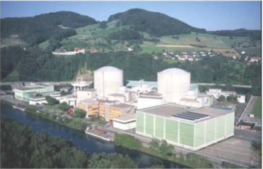
Beznau Nuclear Power Plants (KKB 1 & 2): Two identical two-loop pressurized water reactor units (Westinghouse design). Start operation in 1969 and 1971.
