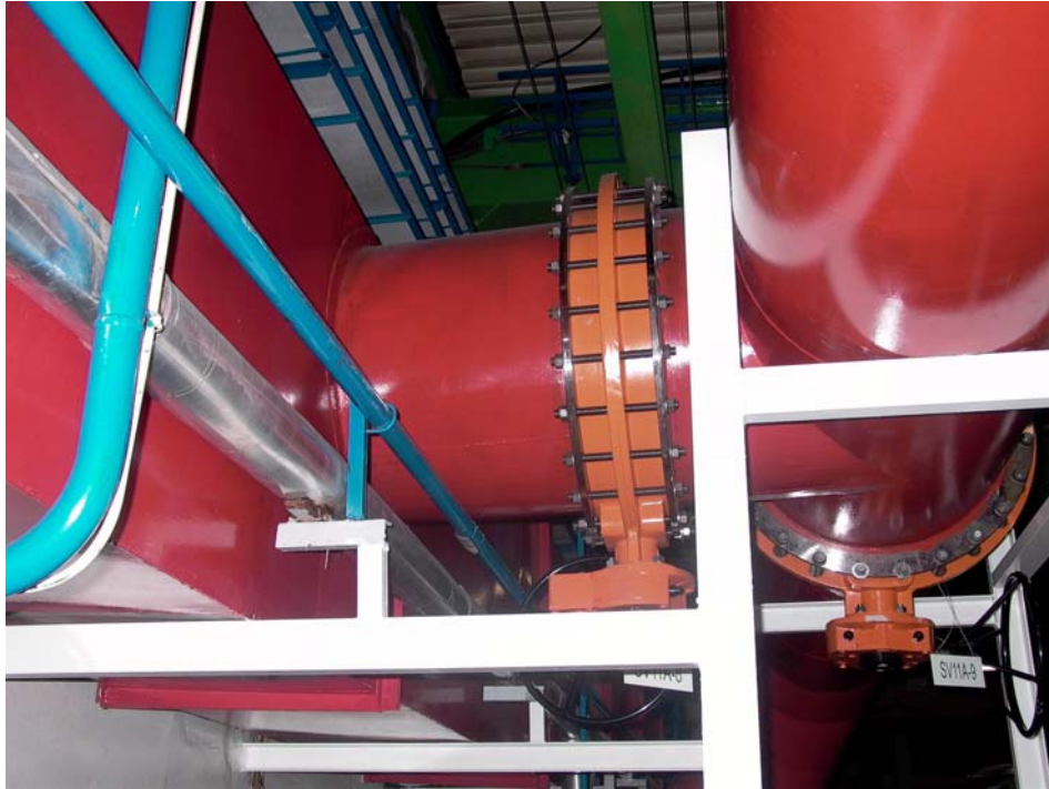
Fig. 7: One part of the modification of air exhaust systems from reactor hall
