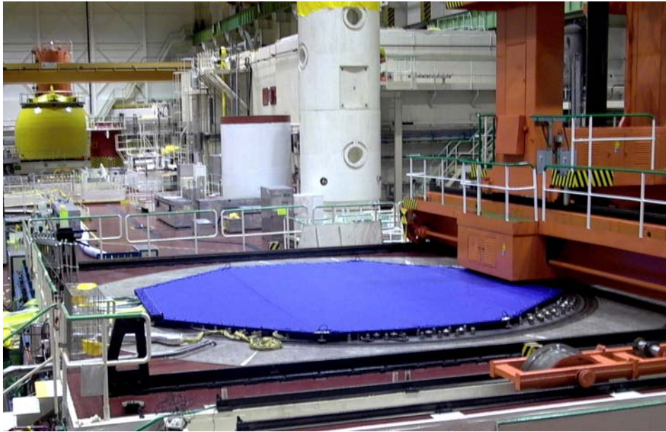
Fig. 3: Blue plastic of the lid, the part of the red refuelling machine and yellow cover of the reactor in the back
