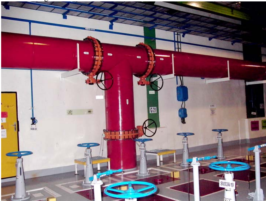
Fig. 4: The modification of air exhaust systems from reactor hall
