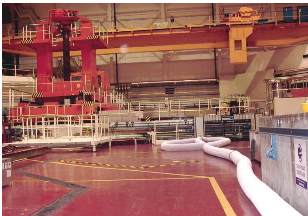
Fig. 2: The example of plastic hose just after its disconnection from the upper part of the control rod drive
