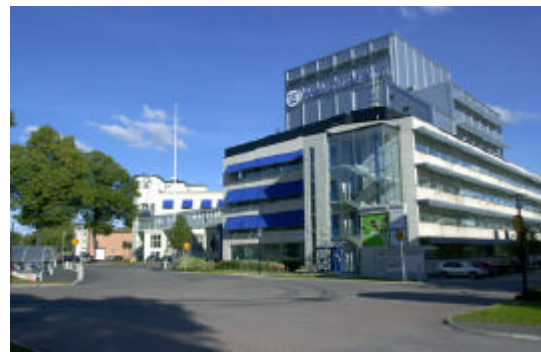
Westinghouse Atom Global reactor services
