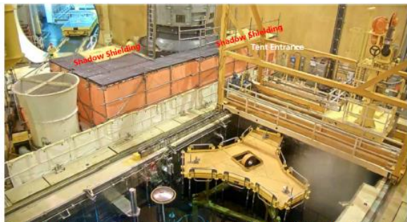
Overview of tent showing tent entrance and extent of tent roof "shadow shielding"
