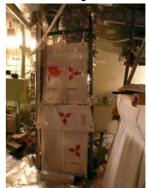
This simplified, portable shielding was used near the RCP motor during its inspection in the ongoing outage (the 2008 outage) for Unit 4. The result was that the dose under the environment where the dose rate is normally about 0.1mSv/hr was about 0.03mSv/hr.
