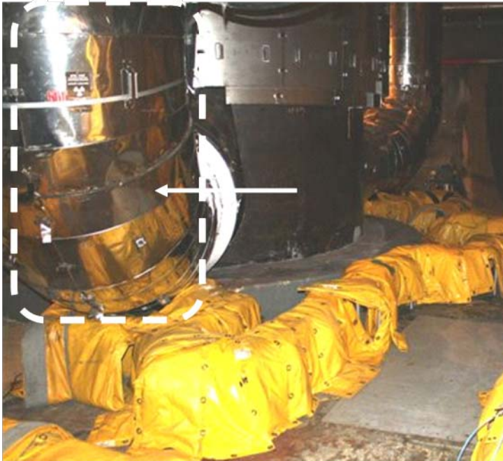
28" OD reactor coolant pump suction piping
