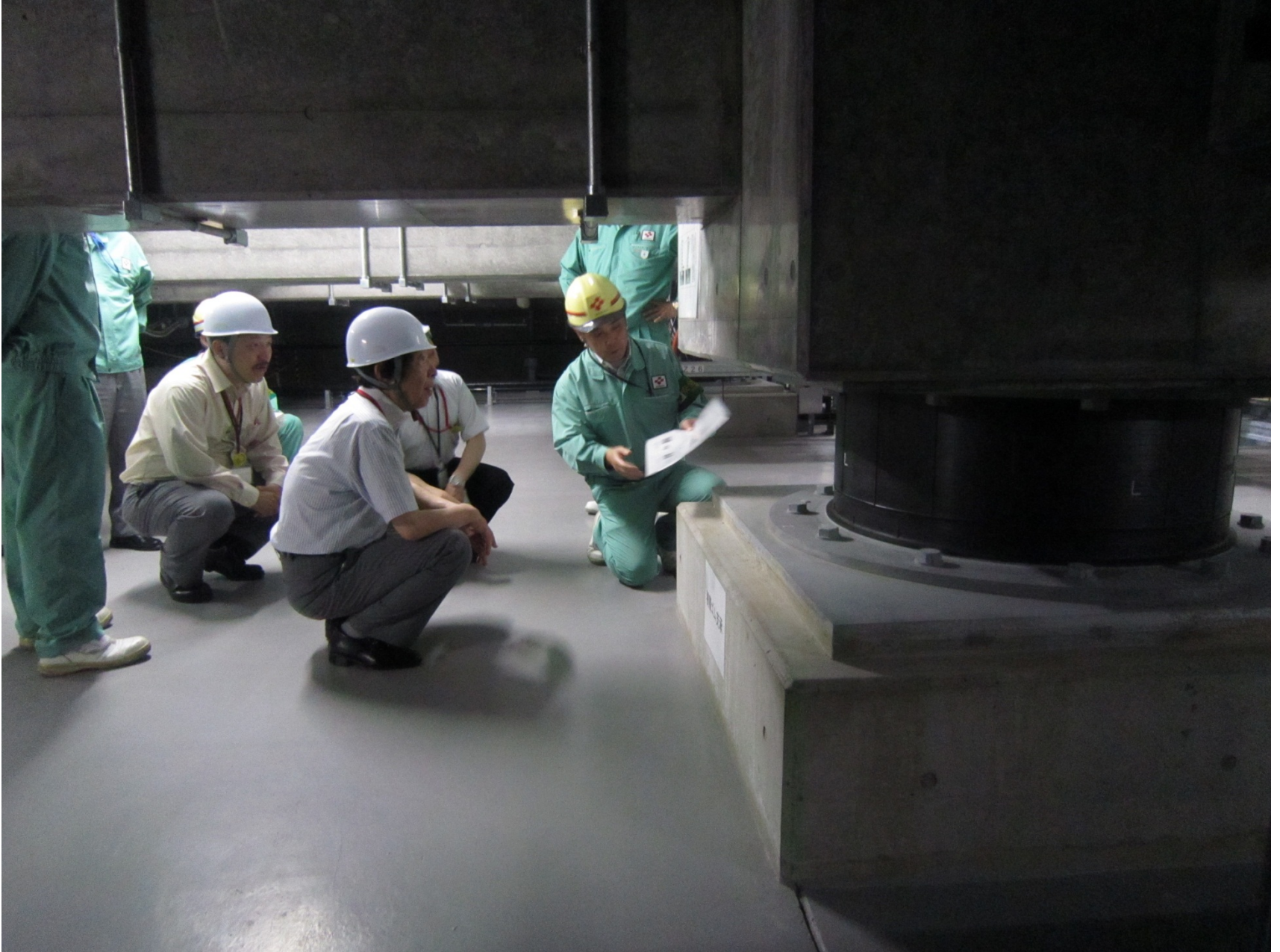
Anti-Seismic Rubbers under Main Office Building at Ikata NPS on Aug 2012
