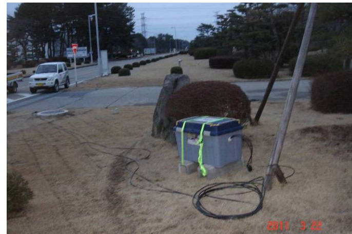
Portable monitoring post at main gate
