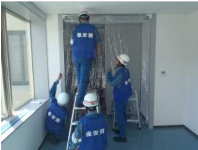
Training to suppress contamination at emergency response room
