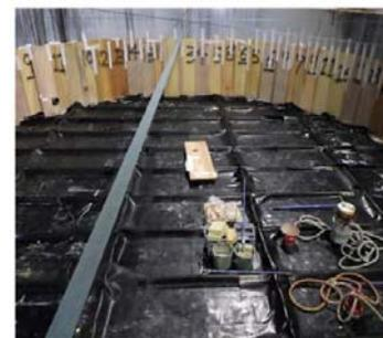
A rubber sheet (to shield radiation from the bottom)
