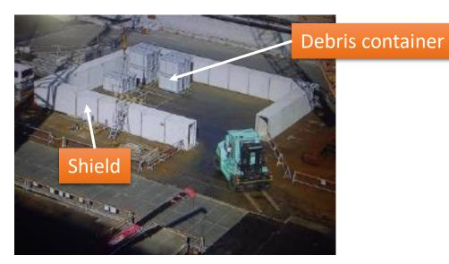
The high-dose container containing the debris from the rooftop of the Unit 3 T/B was placed in the temporary storage area
