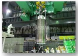
On Dec.22/2014, spent fuel was removed from the SFP of Unit 4, which had suffered a hydrogen explosion as a result of hydrogen backflow from a shared stack with Unit 3, despite the reactor being shut down
