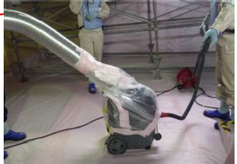
disc grinder with a suction device
